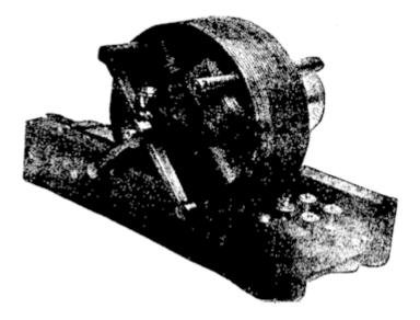
One of the earliest of induction motors. Although it weighed only a little over 20 pounds, it developed 1/4 horse-power at a speed of 1,800 revolutions, a performance considered remarkable at the time.
